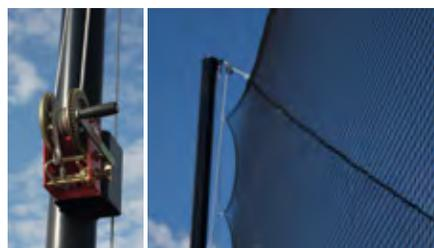
**Lifting winch, top pulleys** and **support cables** make raising and lowering the netting an easy task from the ground.
