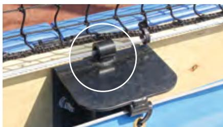
Pads in place, **In-Line Backstop Net** is installed, anchored by the net cable running through the **slide-over post bracket**.
