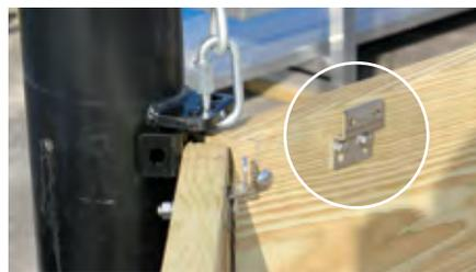
Stainless steel **mounting brackets** and **Velcro wall plates** are added in preparation for adding Wood-less Pads.
